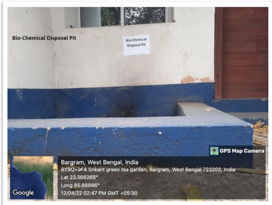
Bio-Chemical Disposal Pit
