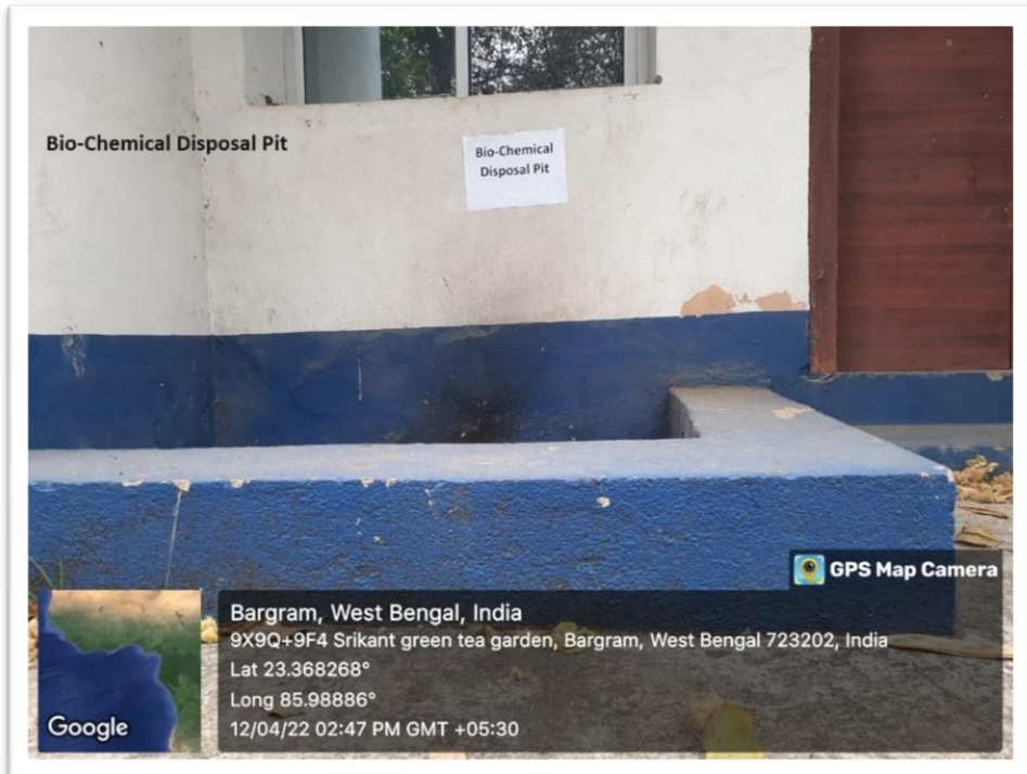
Bio-Chemical Disposal Pit
