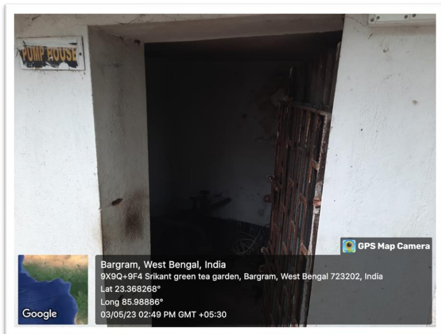
Pump House of Bore Well
