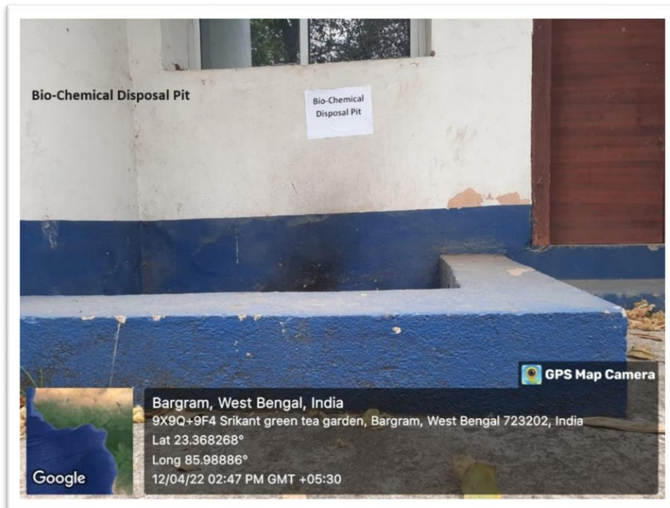
Bio-Chemical Disposal Pit
